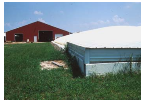
Anaerobic digester downslope from the dairy barn, Haubenschild farm, Princeton, MN. Manure flows from this digester in about 20 days to a holding lagoon where digested manure is held until field-applied in the spring or fall.
