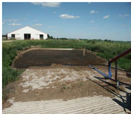
A typical manure lagoon. Manure enters the lagoon directly and is not digested. Depending on conditions, these lagoons may or may not emit unacceptable odors, and methane is not utilized.
