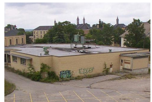
Fig. 2: Future site of Traverse City’s FID Source: Dansby, 2012
