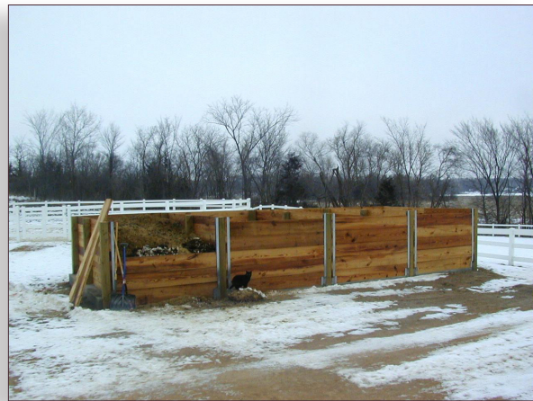
Figure 1. A manure storage bin used for composting. Note slats can be added to front for increased storage.
