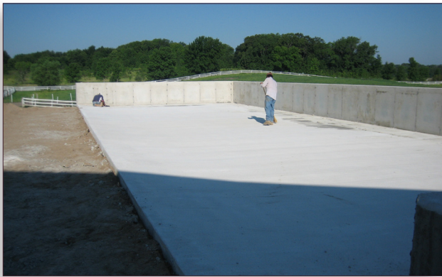
Figure 2. Concrete manure storage pad
