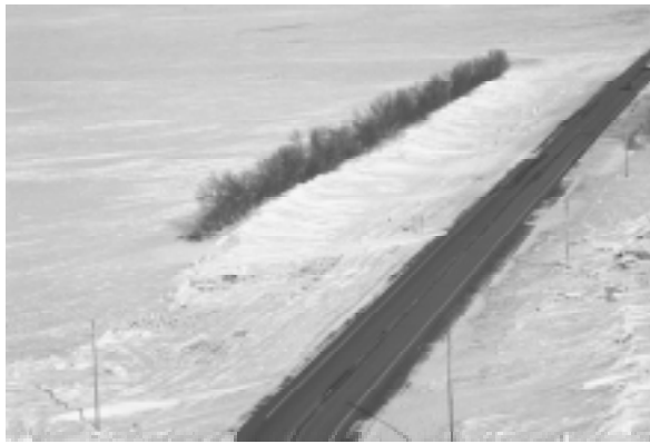
Figure 1. This green ash windbreak was planted too close to the roadway to be effective.
