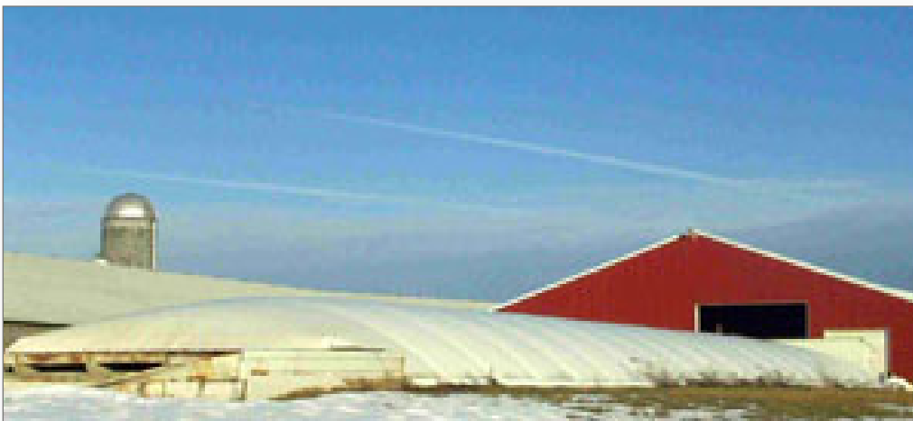
Figure 7: Aerobic digester on Minnesota farm. Credit: The Minnesota Project
