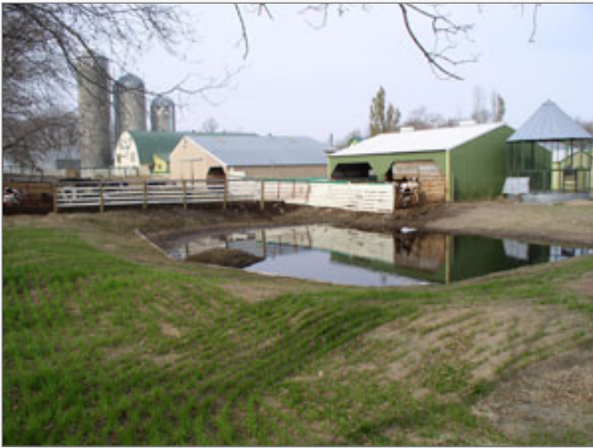
Figure 2: Newly constructed catch basin below an open lot. Credit: Dale Walz, Stearns Co. MN
