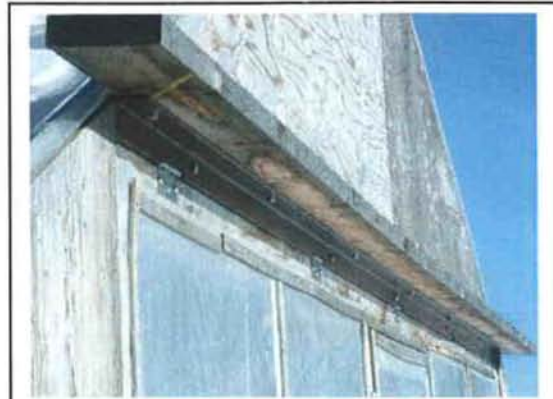
Figure 6. End wall after reinforcement.
