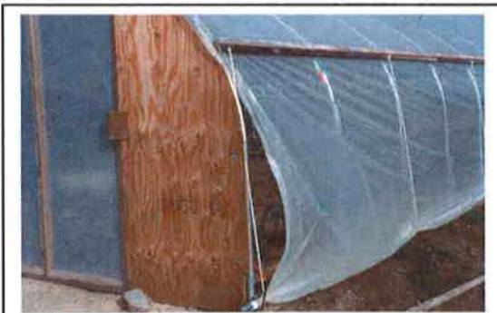
Figure 1. Before corner plastic was attached.
