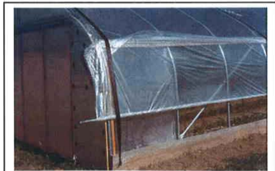
Figure 2. After corner plastic was attached.
