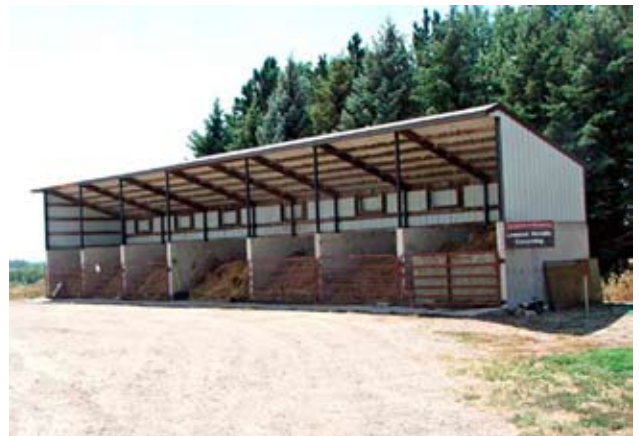
Compost facility at the Research and Outreach Center in Morris. There are seven bins, each bin is 12ft deep x 10ft wide with 6 1/2 ft. concrete side walls.
