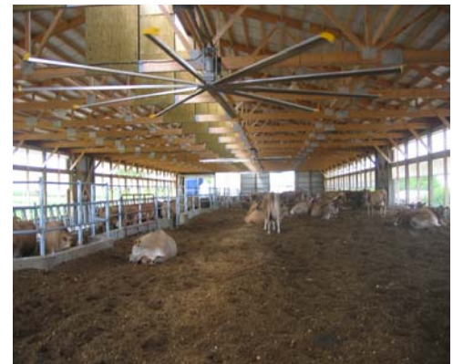
Ceiling fans may be necessary to provide adequate ventilation in the compost dairy barn during the warm summer months.
