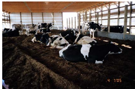
An example barn with 4 foot concrete wall separating the feed alley and the composted bedded pack area.
