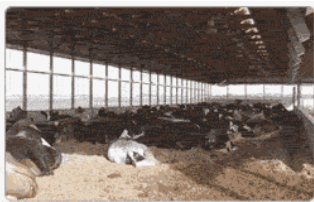
Minnesota Compost Dairy Barn
